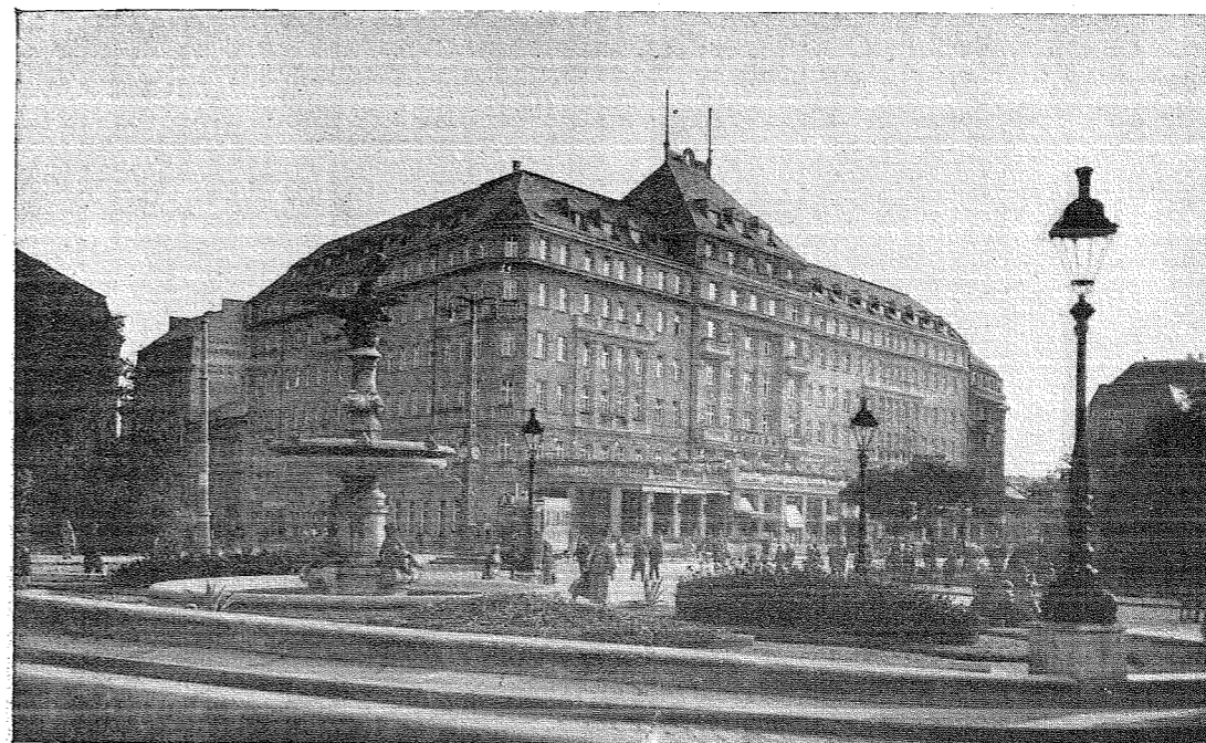
Hotel Savoy-Carlton po prestavbe.
