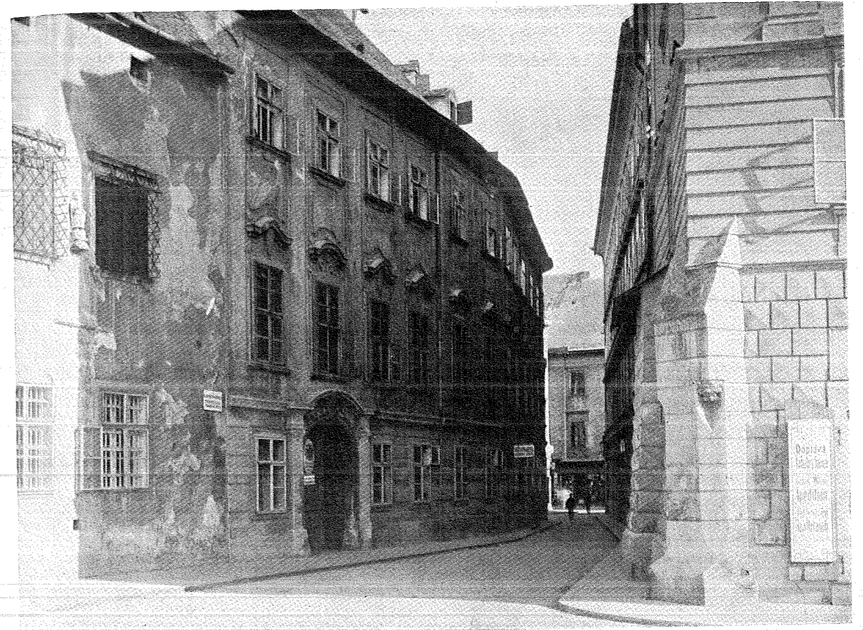
Fassade des Apponyihauses.
